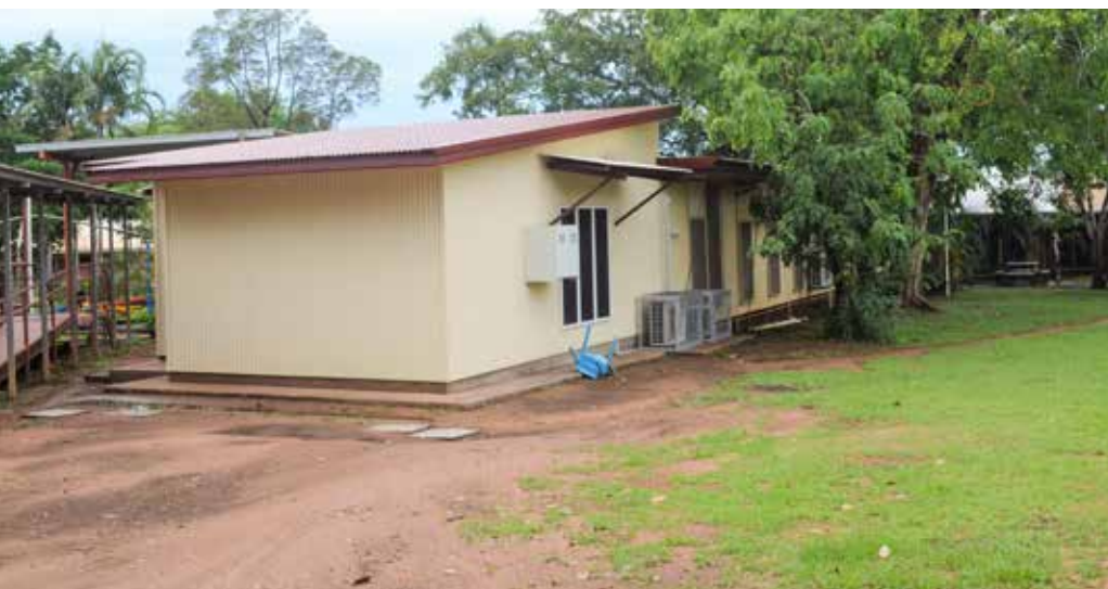
Image: Pirlangimpi New Classroom
